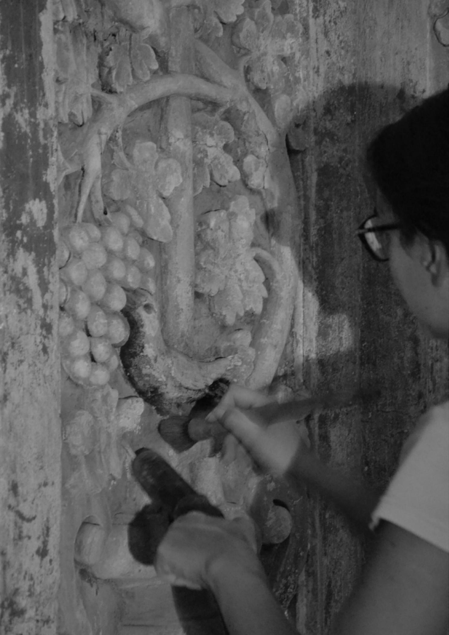
relative humidity within the church was the main cause of damage including micro-decohesion, disintegration of the stone structure, lifting, detachment and losses of fragments of the paint and gilding film, blooming, staining and encrustations. Another detrimental effect caused by the movement of soluble salts was extensive blanching on the gilt and painted surface of the walls.
