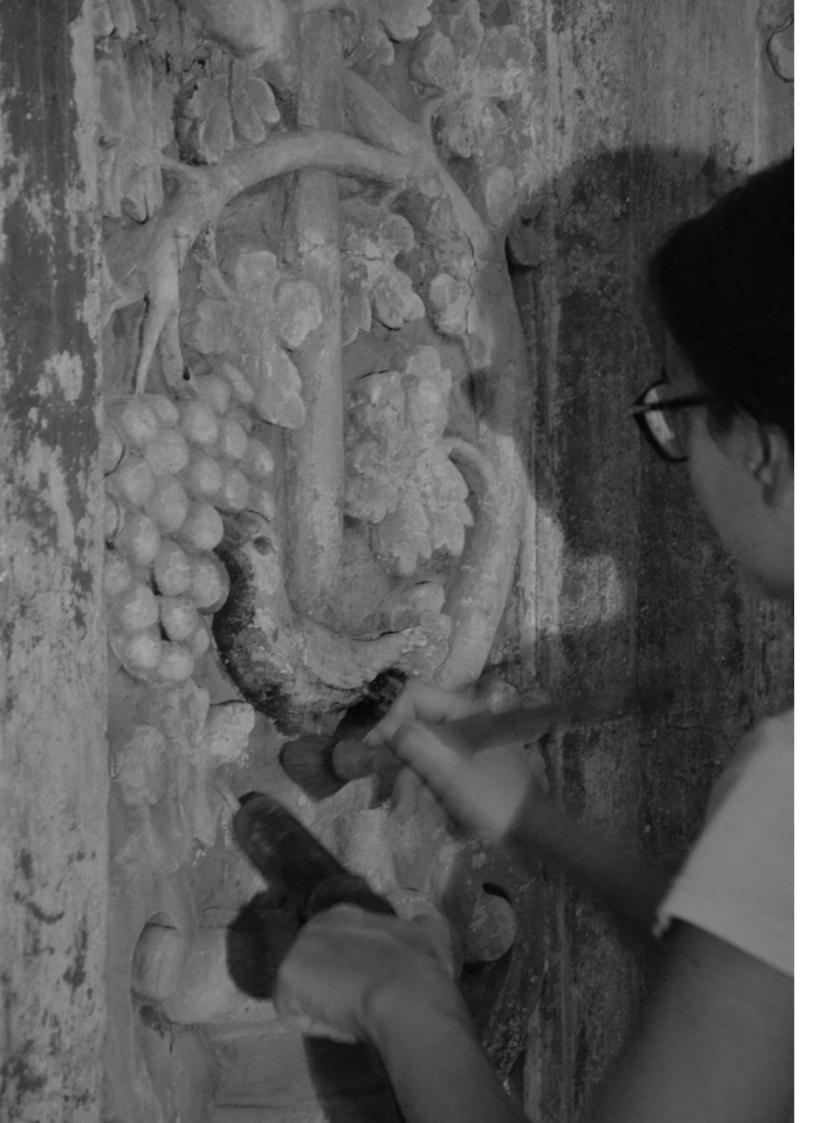
relative humidity within the church was the main cause of damage including micro-decohesion, disintegration of the stone structure, lifting, detachment and losses of fragments of the paint and gilding film, blooming, staining and encrustations. Another detrimental effect caused by the movement of soluble salts was extensive blanching on the gilt and painted surface of the walls.
